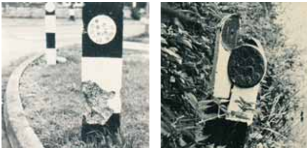
Vergemaster replaced old fashioned concrete and timber posts.
