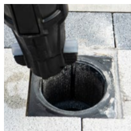
3. Bollard can be removed easily
